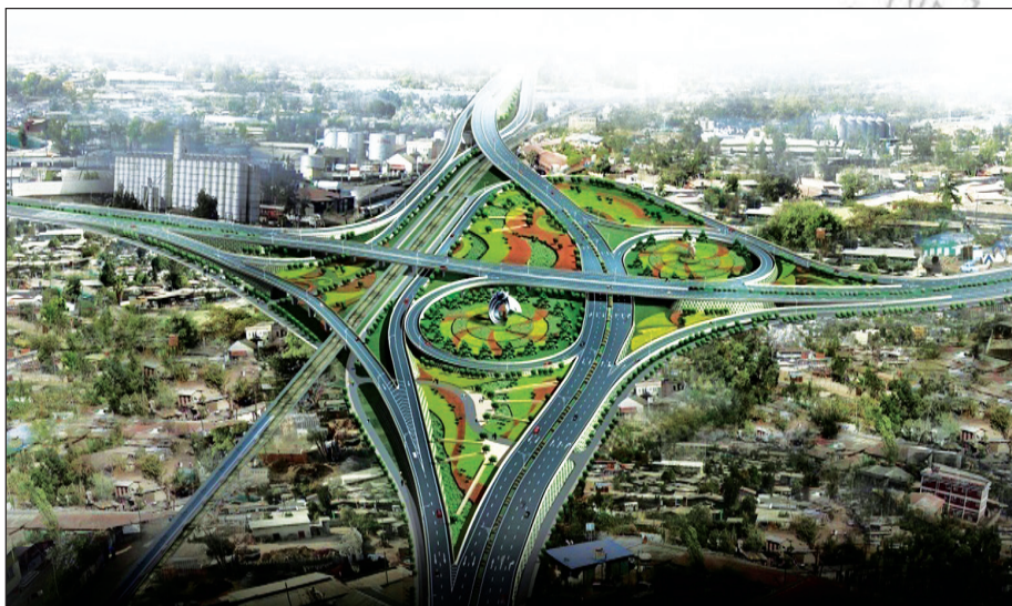
Figure 3.11 Addis Ababa Gotera Interchange Ring Road
